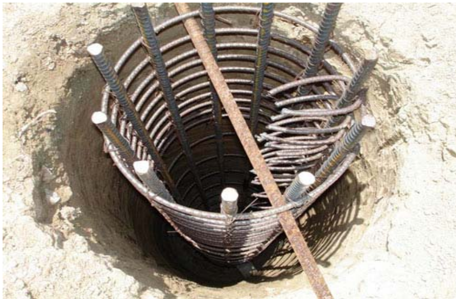
Cast-in-Place Concrete Piles
